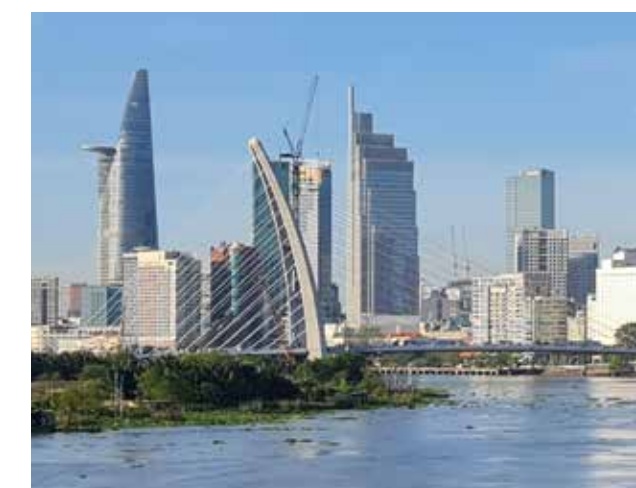
Thu Thiem Bridge The Thu Thiem Bridge 2 main structure spanning 1.5km was completed in December 2021.
